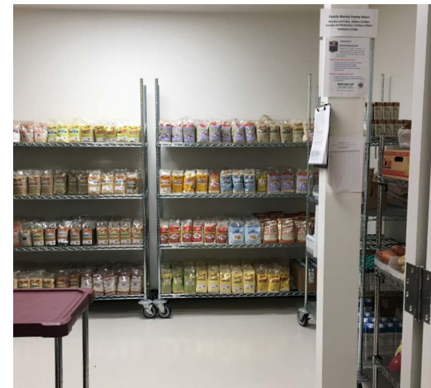
Community Pantry - Example of Dry Storage Room at Providence Milwaukie's Community Kitchen
