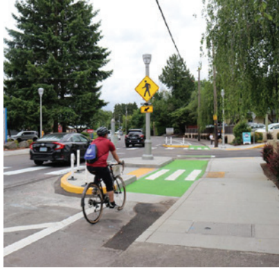
Protected bike lane and highlighted pedestrian crossing at intersection in Portland, Oregon
