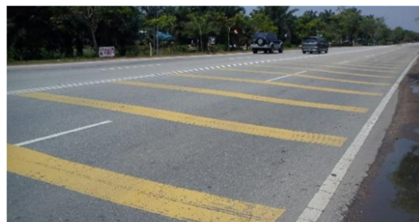
FIGURE 1. Typical transverse rumble strips in Kluang-Batu Pahat Road FT050
