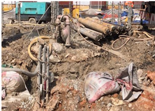
FIGURE 3. Grouting work
