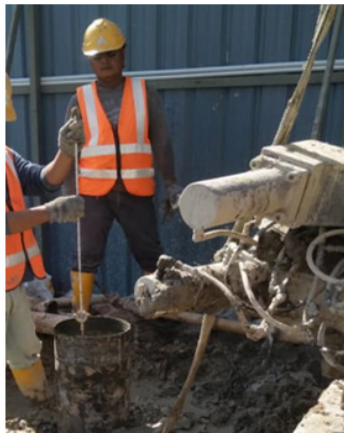
FIGURE 2. Installation of casing pipe
