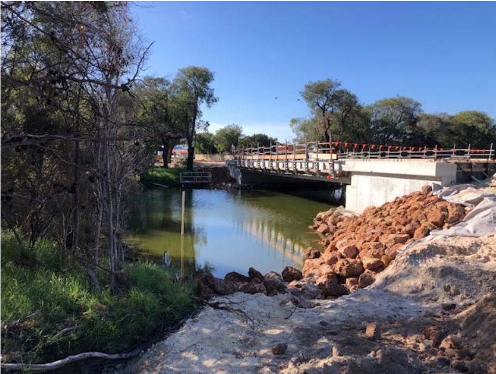
Western side of bridge
