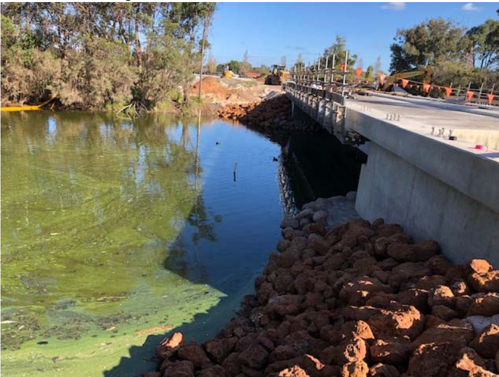
Eastern side of bridge
