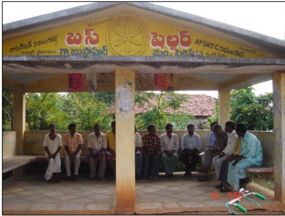
Picture 3. Constructed bus shelter under EPA in Bussapur village
