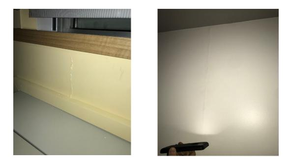
Figure 3-5: Sample of actual damages (cracks) on prefabricated individual modules caused by the transportation-induced forces
