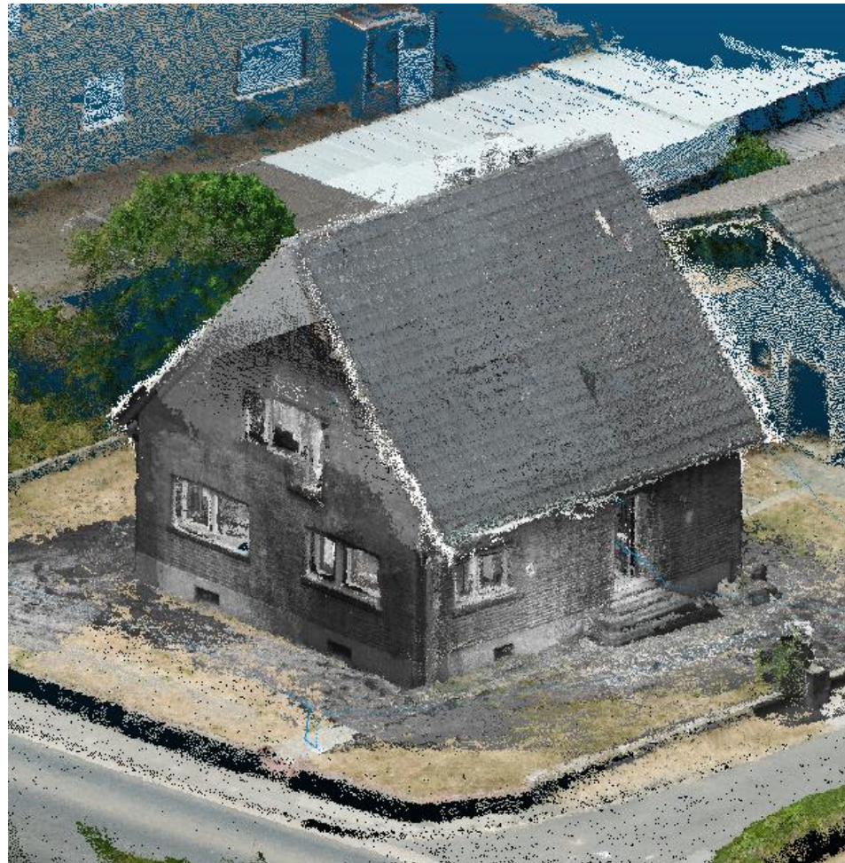
Figure 10. Complementary 3D reconstruction from UAV imagery (colored parts inclusive of the gray roof) combined with IPS on-ground derived point cloud (ground surroundings and building walls shown in grayscale).
