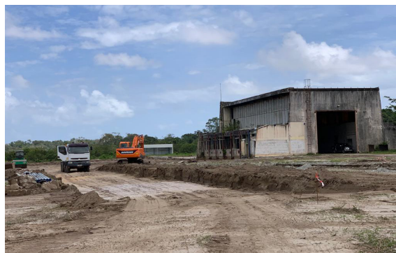
Figure 9 : Civil work around the CALLISTO VPH
