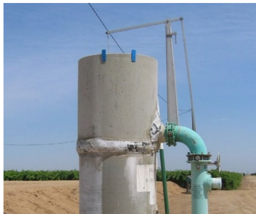
Figure 3. Early float mechanism on a turnout at Delano-Earlimart Irrigation District, discharging into a reservoir. This lacks features such as an upstream manual adjustment butterfly valve, pressure relief valve, and vacuum relief valve.
