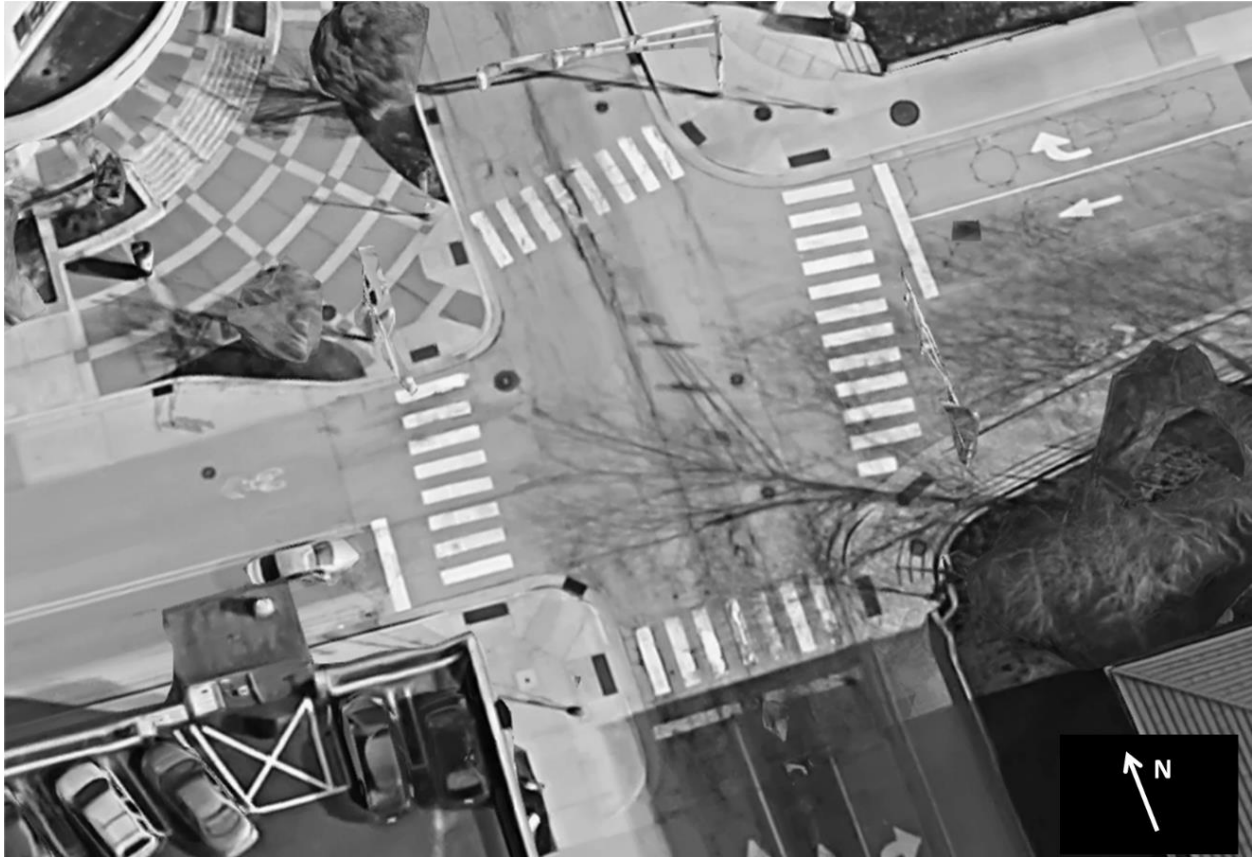
Figure 4. Observation Location 3. Source: Google Earth coordinates 40°25'38"N 86°55'00"W.
