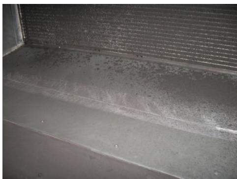
Figure 3.27. Test run 2C; lower pressure drop measured (2014).
