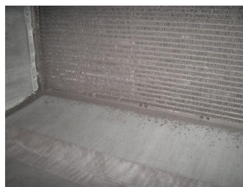
Figure 3.30. Test run 2E; lower pressure drop measured (2015).
