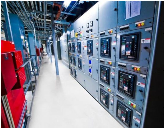
Figure 4: Data center for processing data communication
