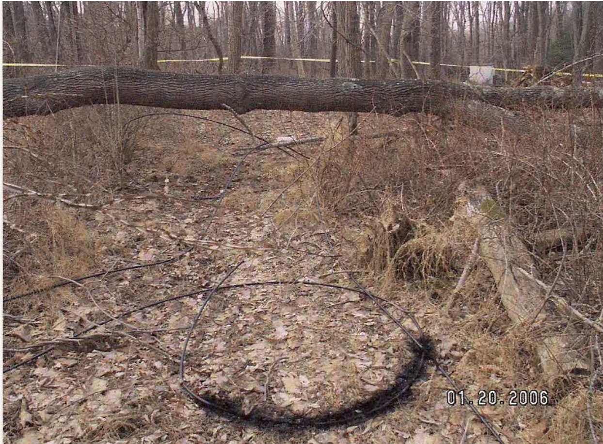
Figure 7: Fallen tree with broken power lines and stretched cable lines.
