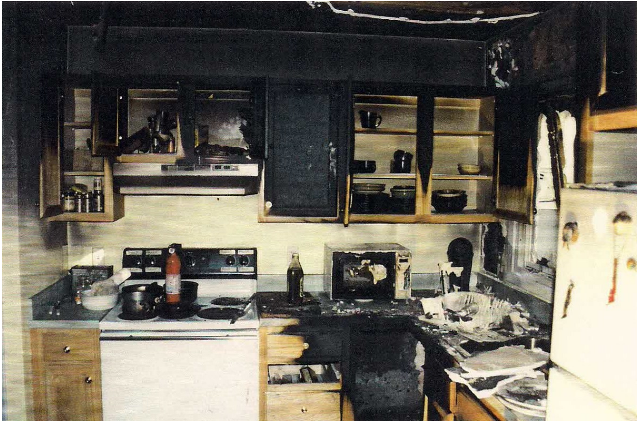
Figure 4: Damage of fire caused by fridge wire under microwave cabinet was small. However, the owner died of smoke inhalation. NOTE: fire extinguisher on top of stove, un-used.
