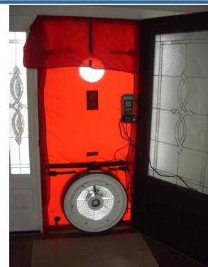
Measuring Air tightness with blower test
