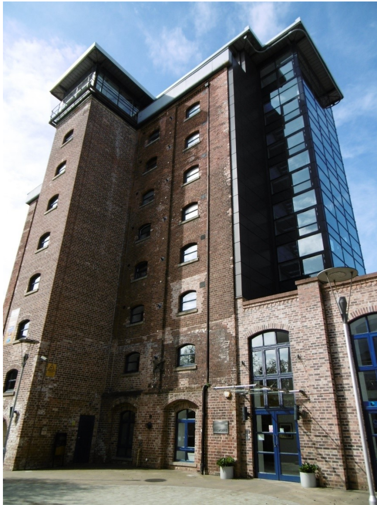
Figure 1: Sugar Bond House, Class 2 Listed Building Photograph by author
