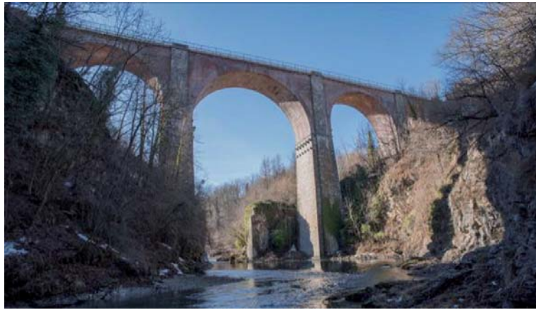
Fig. 1. The Olla bridge: view from the Stura river.
