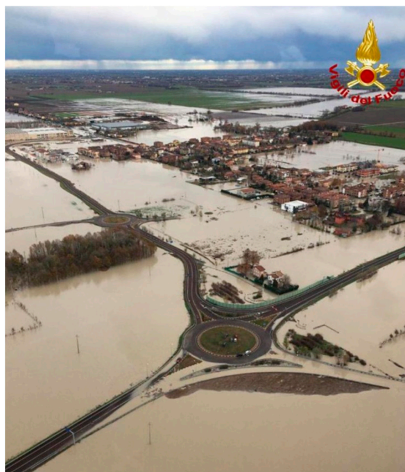
Figure 3. Picture of the flooded area of Nonantola (courtesy of the Italian National Fire Corps).
