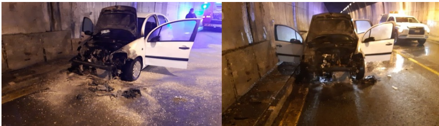
Figure 8: Vehicle involved in the event inside the San Rocco tunnel. (Source: Strada dei Parchi S.p.A.)
