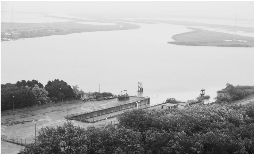
FIGURE 14.16 The dock for barge unloading. Source: Chiara Geroldi.
