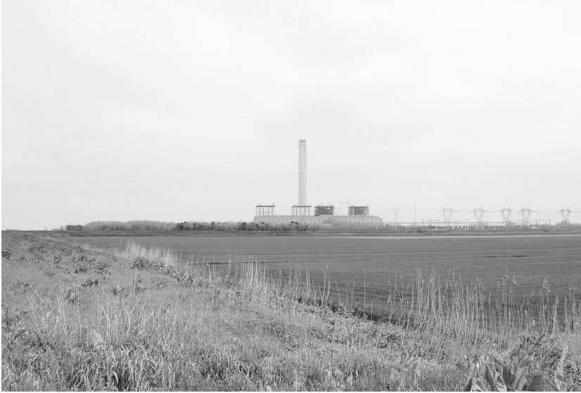
FIGURE 14.13 Porto Tolle power station. Source: Chiara Geroldi.
