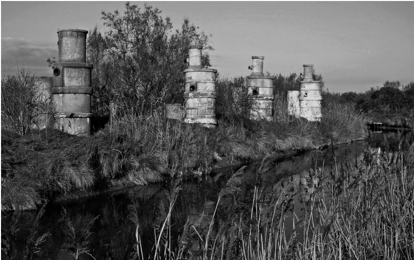
FIGURE 14.9 Abandoned methane gas extraction wells in Ca' Pisani (Porto Viro, RO). Source: Moreno Bonifacio.
