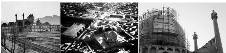
Fig. 9. From left to right: wooden scaffolding for eyvan restoration, photo by Robert Byron, 1933, Courtauld Institute of Art Source Fine Arts Library, Harvard; Aerial view of Shah mosque shows the strengthening that had been applied, 6 July 1937, The Oriental Institute, The University of Chicago; dome strengthening of 1941 by the encircling steel ties system, 2018
