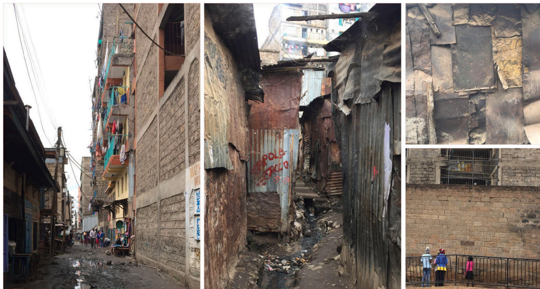
Fig. 16. All images within Mathare DUA taken by the author. Left: Buildings with walls made of bricks. Middle: Buildings with walls made of iron-sheets. Top-right: Iron-sheet wall detail. Bottom-right: Brick wall detail.
