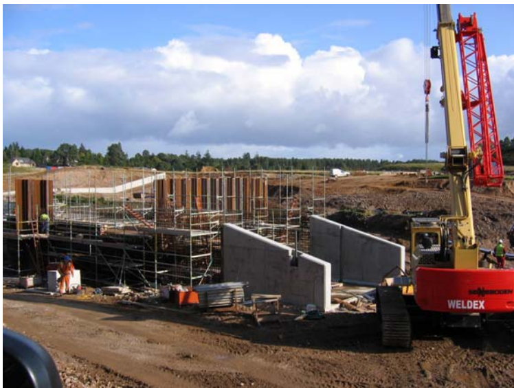
Construction of flood defences at Chapleton Moss, Forres Cost £20 M
