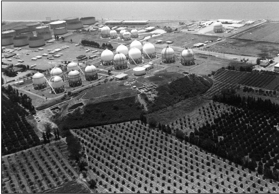
Pl.1. Aerial View of Kinet Höyük with the Delta Petroleum Company Facilities
