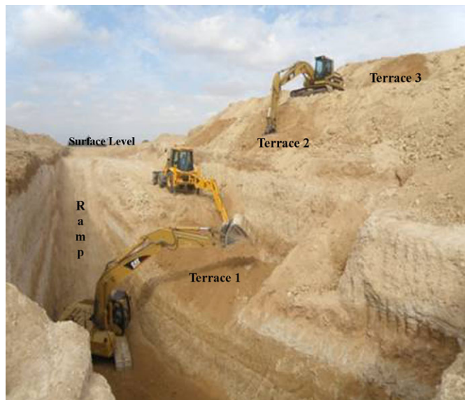
FIG. 3—Terracing method as applied to the soft landform of Akdogan-Lisi Well excavation, in the northern part of Cyprus (2009).
