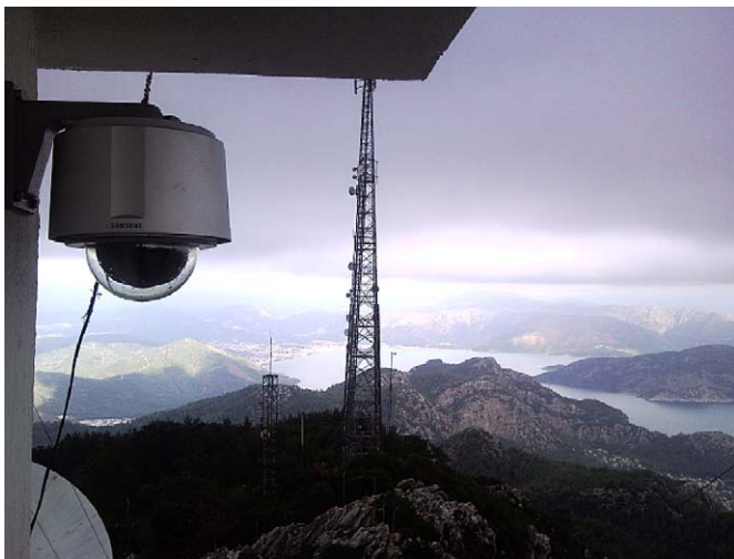
Fig. 6. Samsung analog camera mounted at the watch tower.
