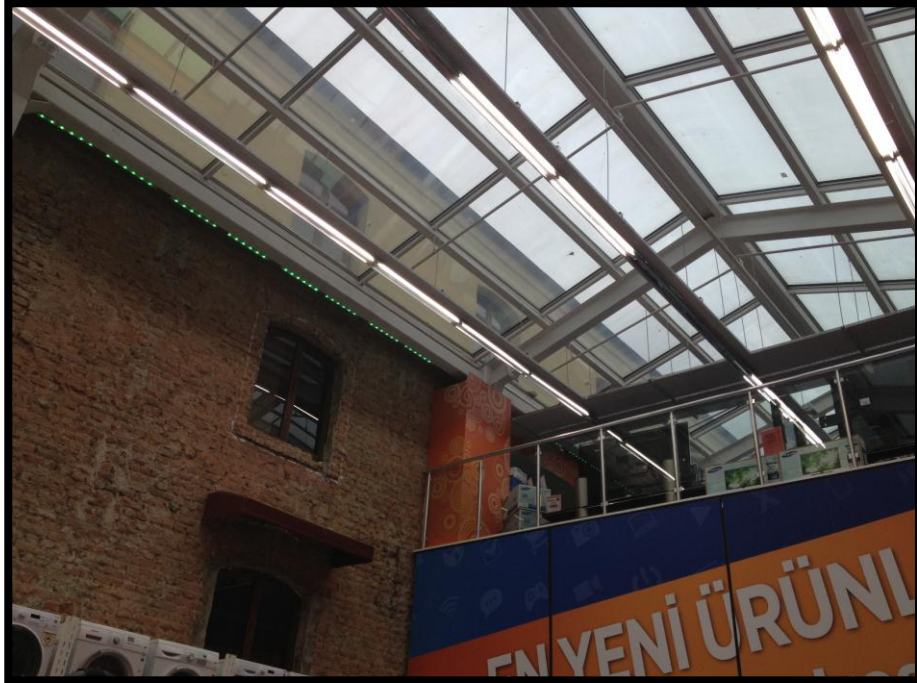
Figure 5.10. C-D Block Interior 34
