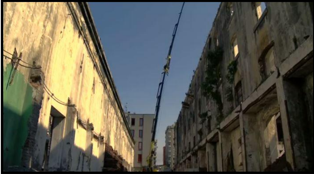
Figure 5.3. Construction Site of The Factory Buildings 27
