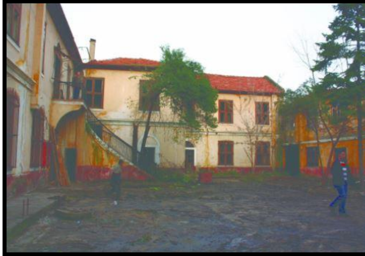
Figure 4.13. A Block Courtyard 14
