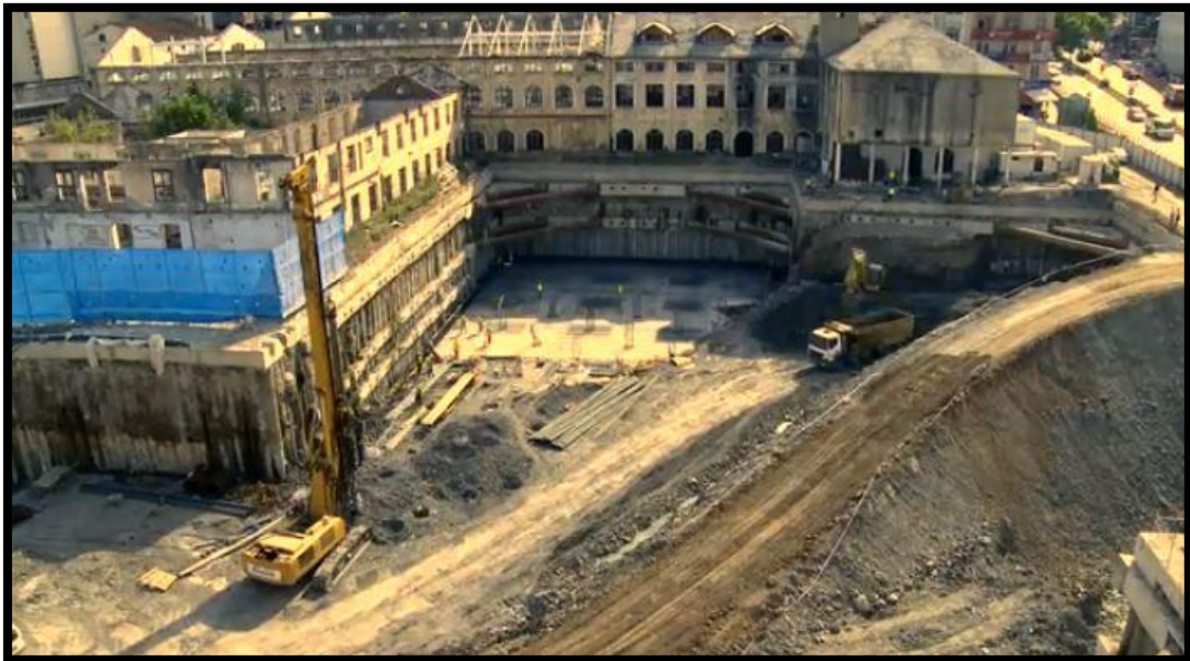
Figure 5.2. Construction Site of The Factory Buildings 26
