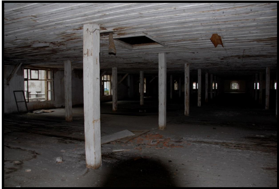
Figure 5.15. Indoors of the Factory – Before Reevaluation 39
