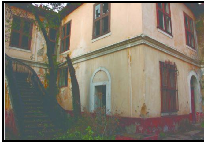
Figure 4.14. A Block Courtyard 15
