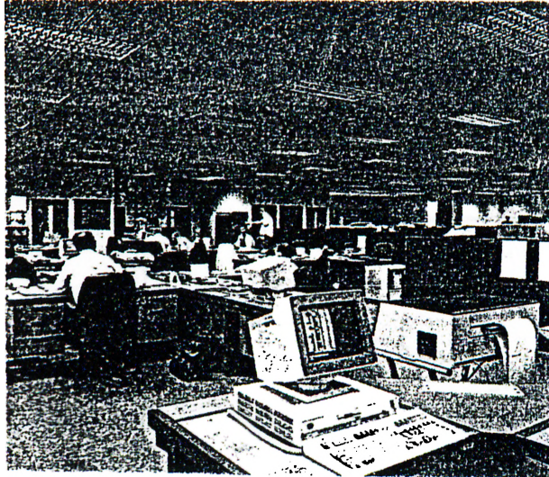
Figure 3.19 Open plan office with downlight installation (CIBSE Lighting Guide: Areas for Visual Display Terminals, 1989).
