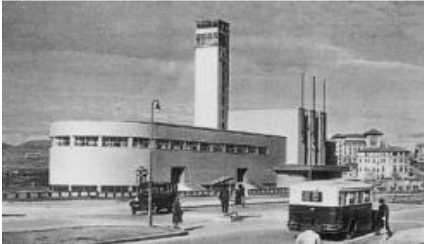
Figure 15: The exterior view of the Balmumcu's Exhibition house (Vanlı,2006: 28)
