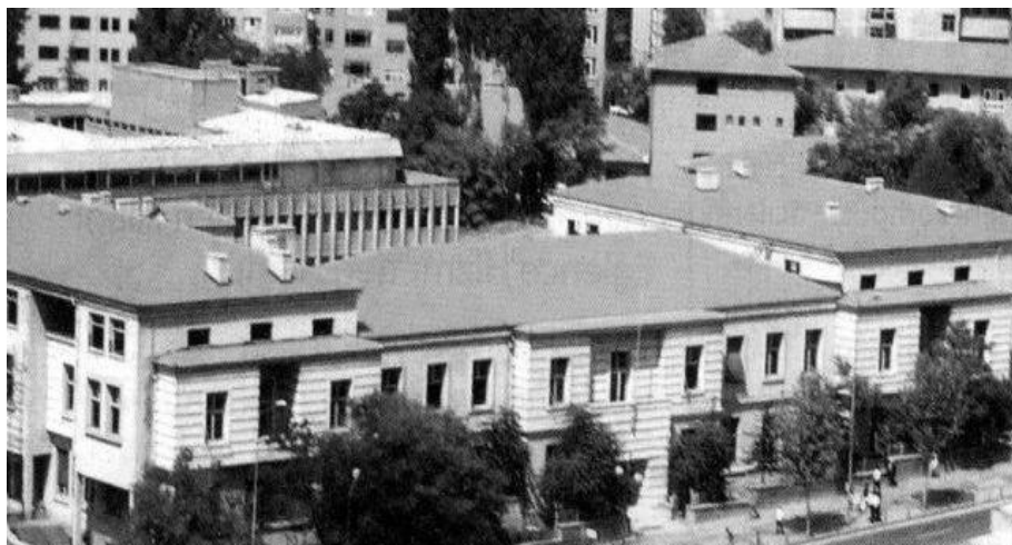
Figure 23: Egli's Court of Finacial Appeals Building in Ankara
