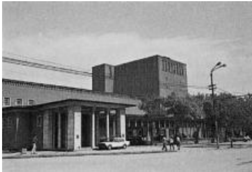
Figure 16: The exterior view of the Bonatz's Opera house (Vanlı,2006: 29)
