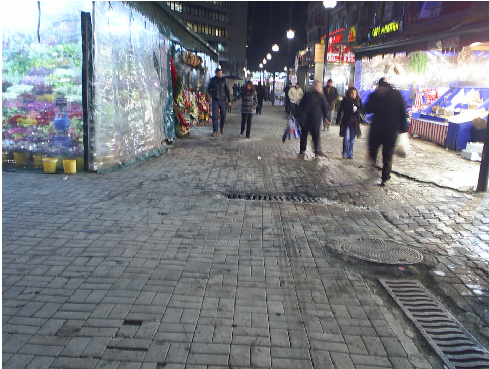
Figure 12.6. Accumulated dirty water of fish shops on distorted sidewalks (March, 2009, weekday evening)
