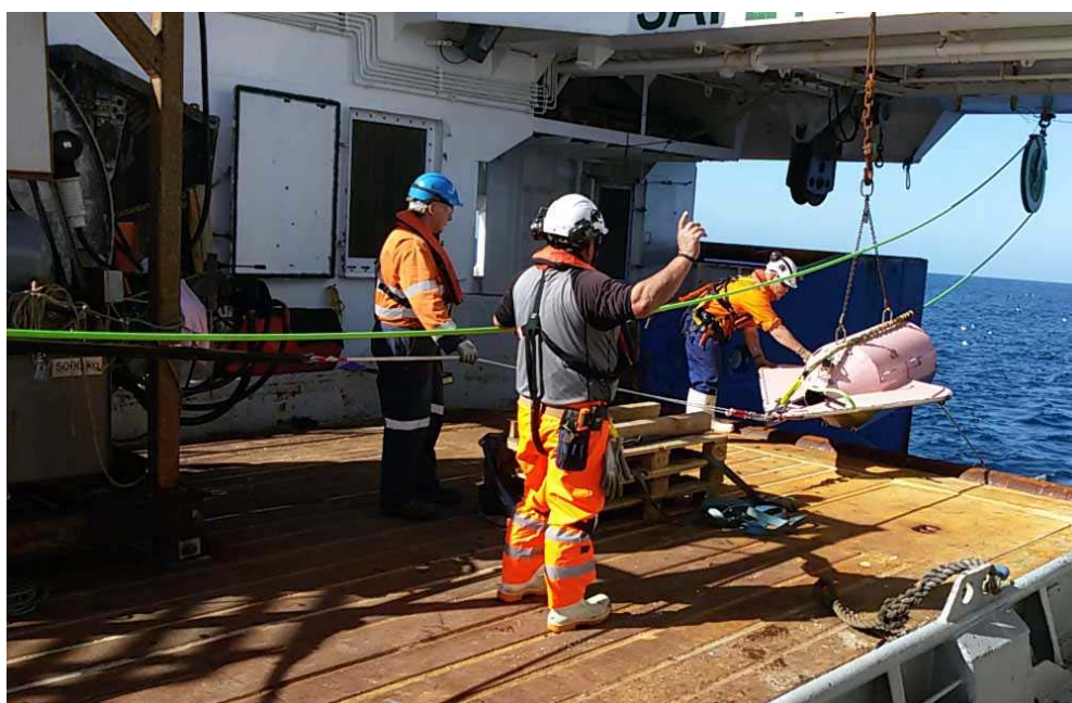
Figure 25: Pig deployment and recovery procedure
