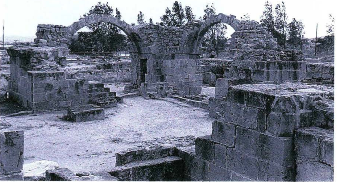
2b Saranda Kolones: vaulting and piers for the undercrofts (photograph by the author)
