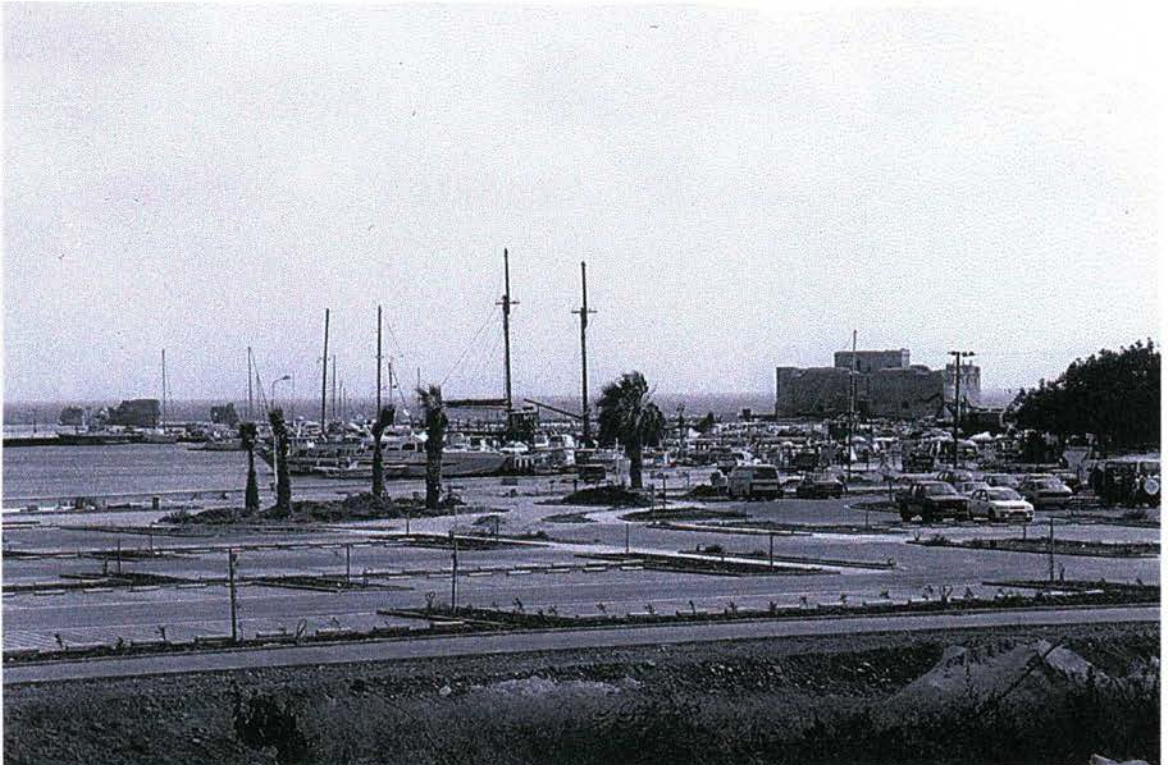
28a Paphos Harbour: Paphos Fort and Harbour Tower are visible (photo by the author)
