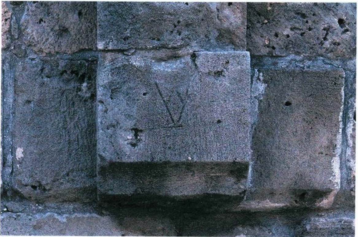
8b Saranda Kolones: mason's mark on the south west pier (photograph by the author)
