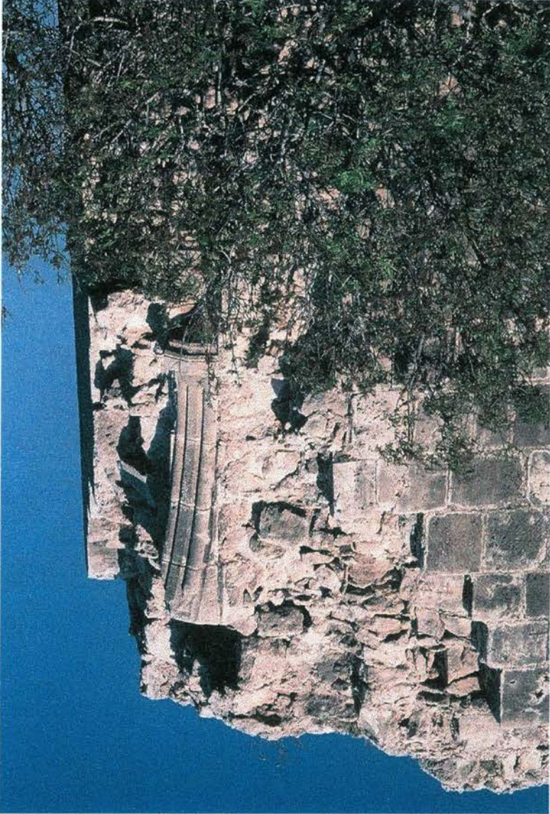
11 Latin Cathedral: detail of vaulting rib (photograph by the author)
