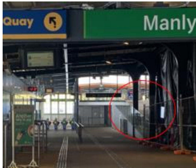
Figure 8 Manly Wharf Ramp
