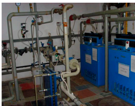
a) hot water boilers of the hot water circuit
