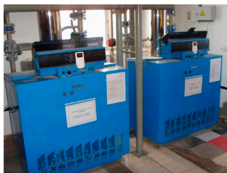
a) hot water boilers of the hot water circuit
