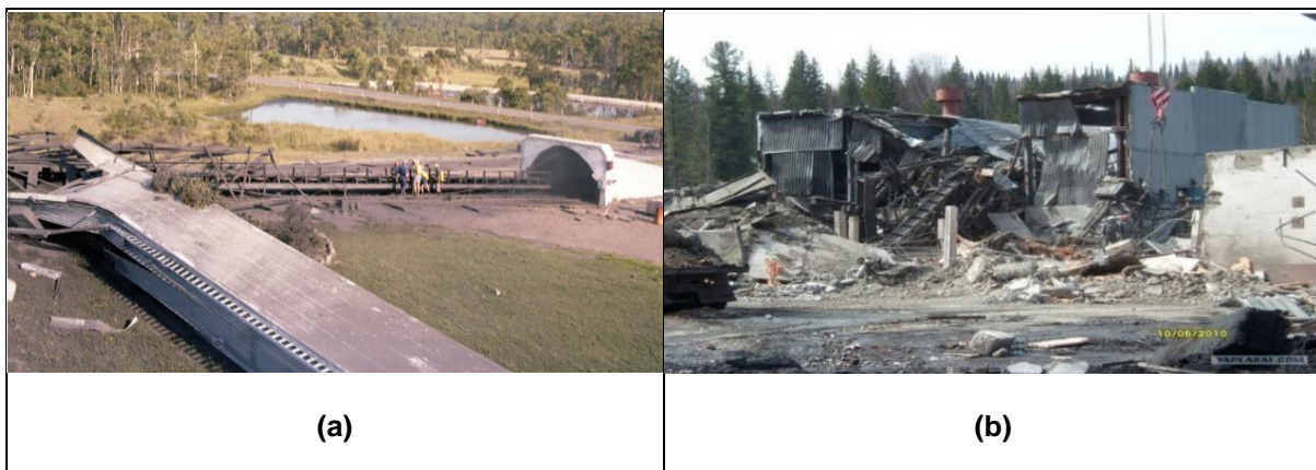
Figure 1: (a) The ventilation shaft of West Wallsend was thrown off by the explosion (Living Histories 2017), and (b) infrastructure facilities were damaged by the explosion in proximity to the Rospidskaya mine entrance (Mine Accident and Disaster Database 2021c)
