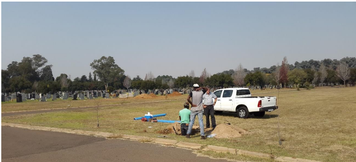
Figure 3-5. Excavation of the 5th groundwater monitoring point.
