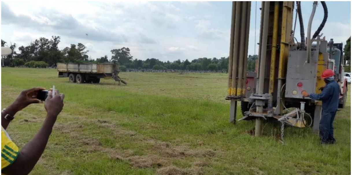
Figure 3-2. Drilling of monitoring boreholes at Fontein Street Cemetery.
