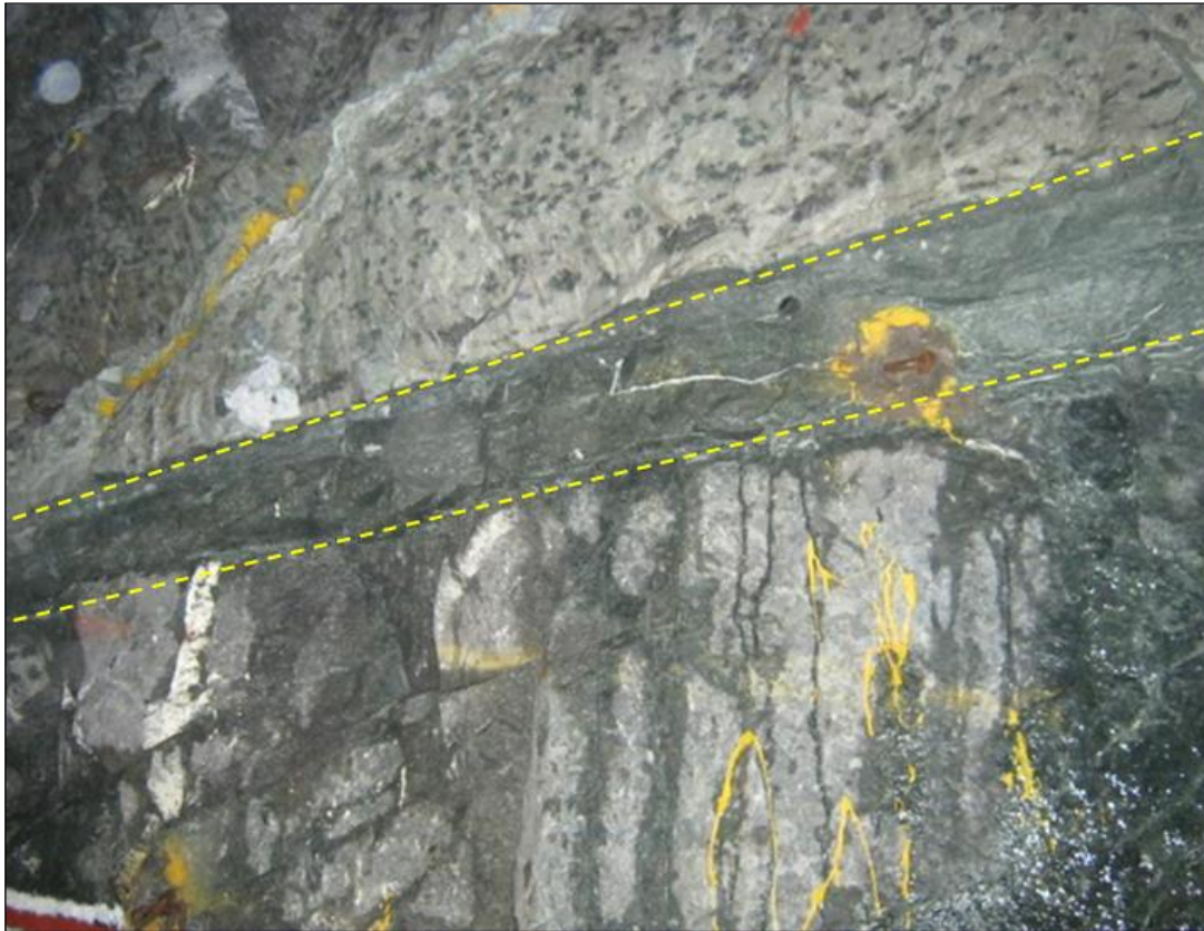
Figure 1.4: Footwall 5/6 shear exposed in an off-reef development excavation (a decline) at an Eastern Platinum Limited Shaft.
