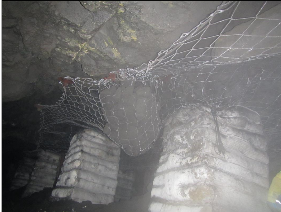
Figure 4.32: Permanent, blast resistant mesh to prevent the unravelling of the alteration zone.
