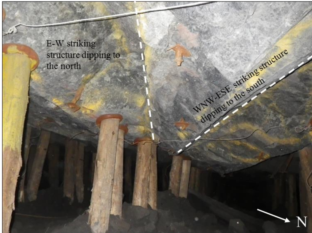
Figure 3.18: E-W and WNW-ESE striking structures exposed in a panel.
