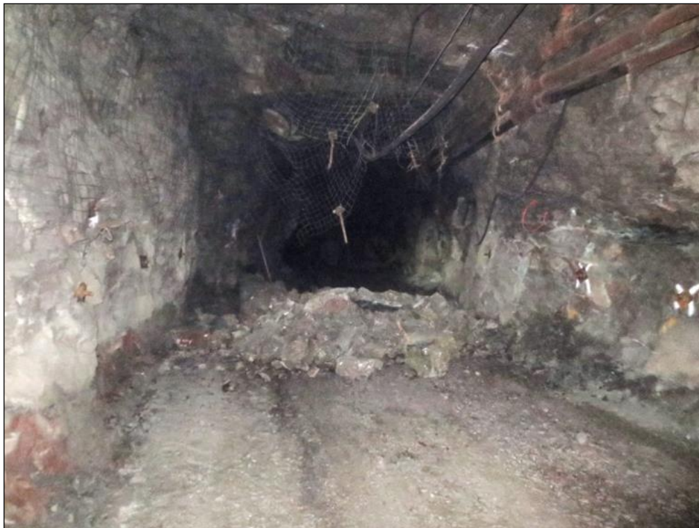
Figure 2.38: Localised fall of ground (More O’Ferrall and Du Plessis, 2017).
