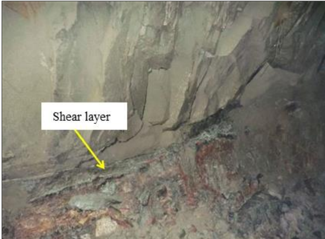
Figure 2.39: Shear layer exposed in the underground workings.
