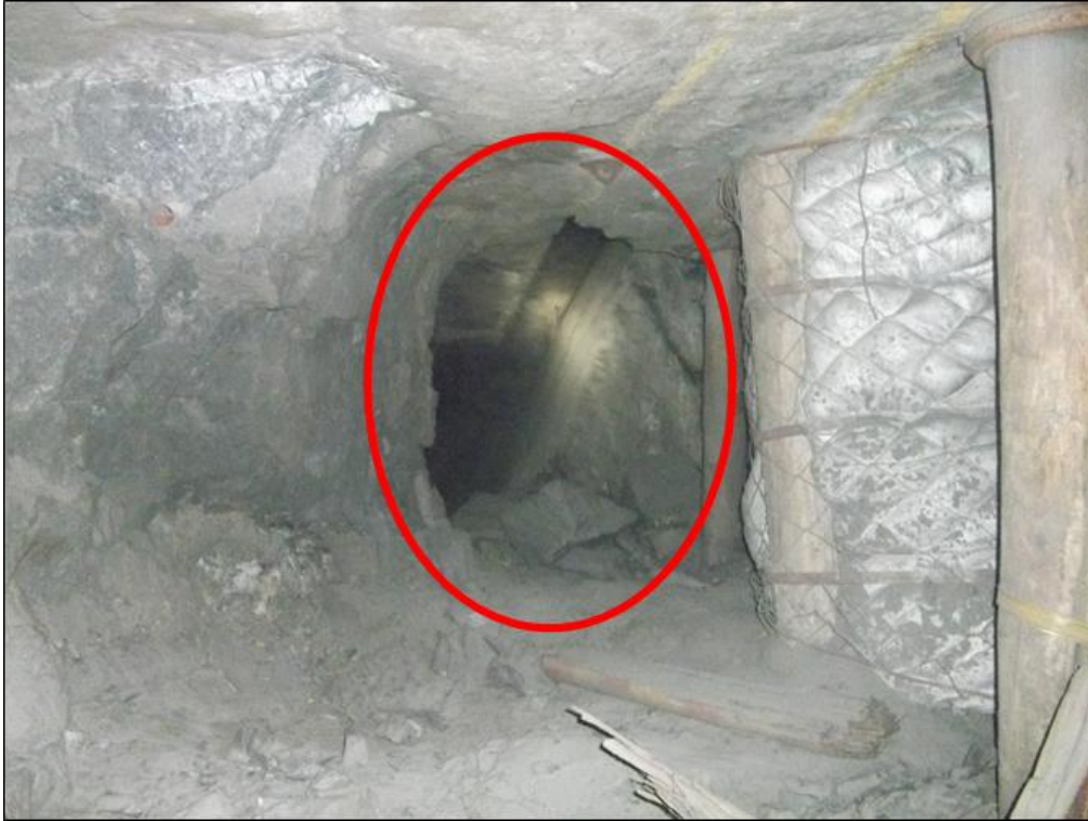
Figure 1.9: Panel instability shown in the red ellipse. The entire panel was affected along a regional large-scale WNW-ESE trending fault structure. Separation occurred at approximately 12 – 15 m in the hangingwall (along the hangingwall 1A/hangingwall 2 contact). The panel had to be re-established.
