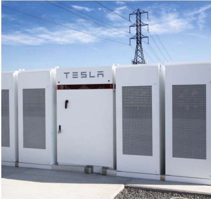
Figure 13. Example Tesla Powerpack System. Source: Tesla (2017, 6).
