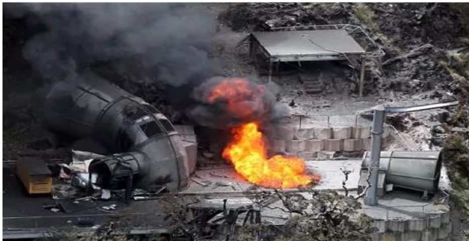
Figure 8: Fire flames coming out the ventilation shaft after the Pike River disaster (The National Business Review, 2013)
