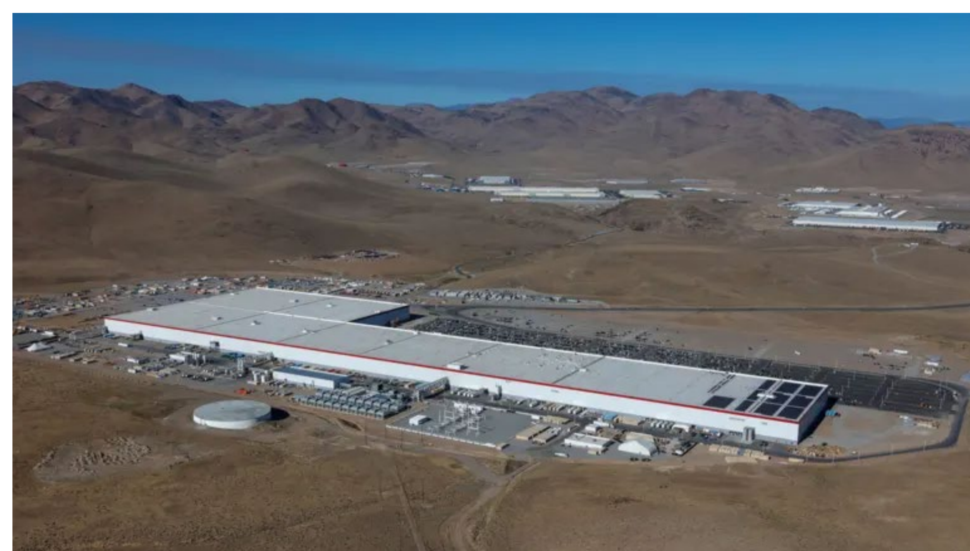
U.S. Battery Manufacturing Plant
