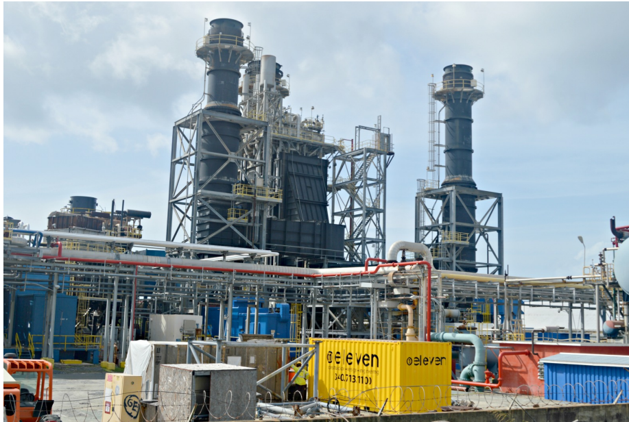
Figure 8. Richmond Power Plant. Photo: VI Consortium.
