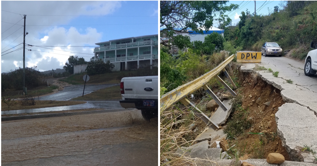
Figure 24. Left: Rainfall in March 2018 causing downhill soil erosion and heavy street flooding north of Christiansted, St. Croix. Right: A washed out road from heavy rains from Hurricane Irma reduces traffic to one lane in the hills above Charlotte Amalie, St. Thomas. Photos: NPS, 2018.
