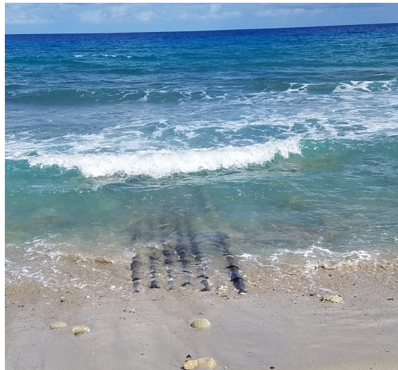
Figure 34. One of the two fiber cable landing sites - North of Fredriksted. Photo: NPS, March 2018.
