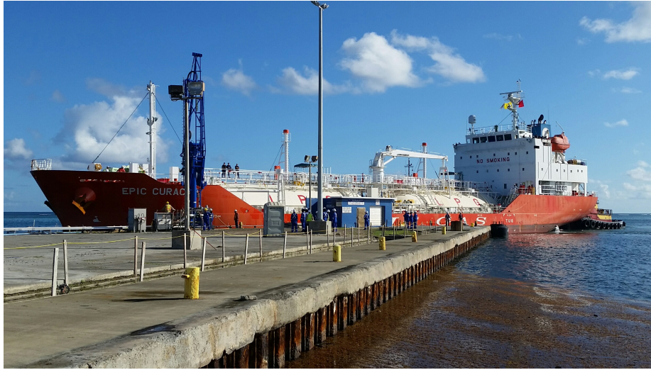
Figure 14. Offloading LPG to VITOL LPG Terminal in Christiansted. Photo: St. Croix Source.
