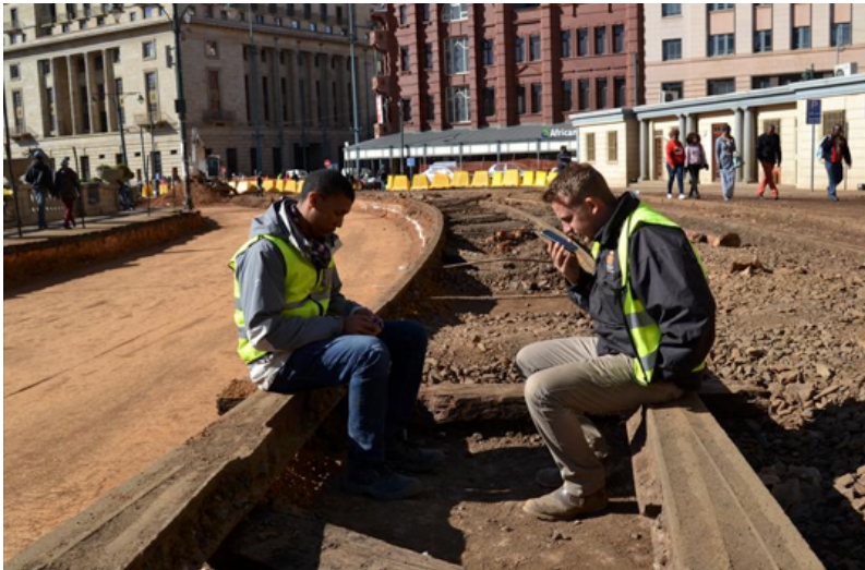
Figure 126: The remnants of the original historic tram tracks were exposed during a construction project on Church Square; the tracks are still in a good condition, as depicted above (Melvin Residence 2014)
