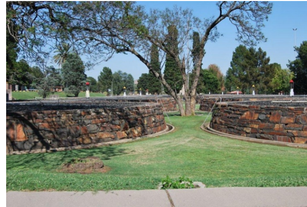
Figure 128: The trickling ponds at the Daspoort Sewage Farm are an example of excellent stone masonry, dating from the 1920s (the Author)
