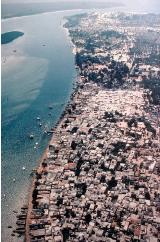
Figure 56: Lamu Old Town Kenya (UNESCO 2001a). An aerial photograph showing the fine-grained urban fabric of Lamu Old Town.
