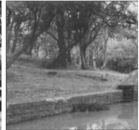
Figure 118: Water structure historic Pretoria - masonry funnel leading to sump at the pump chamber (Panagos 2003)
