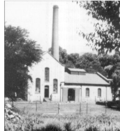
Figure 117: Water structure historic Pretoria - pump station built by the British circa 1898 (Panagos 2003)
