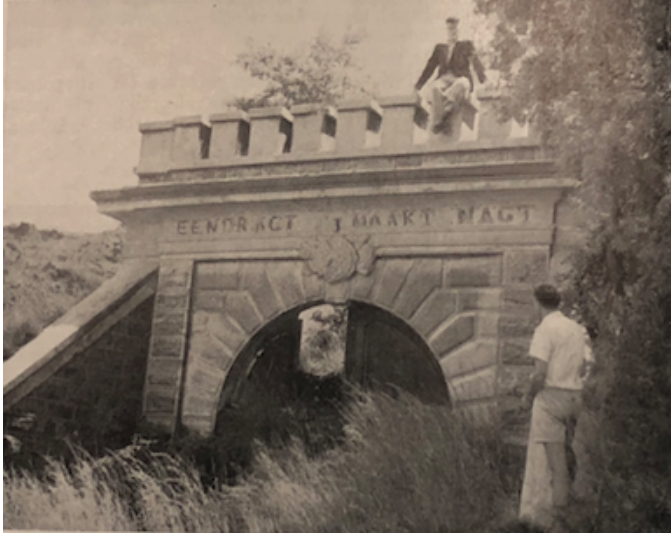
Figure 80: The entrance to Wes Fort at Daspoortrand, Pretoria (Engelbrecht et al. 1955, p. 100)
