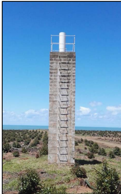
Figure 4.2: Trigonometrical beacon Baton Rouge No 276 on a 6 m concrete block in the northern part of the Amatigulu River mouth.
