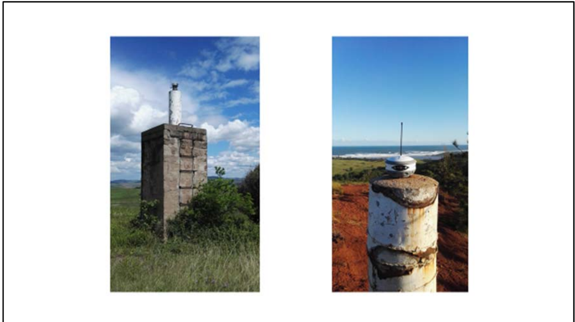
Figure 4.1: Trigonometrical beacon Aloes II (left) and Red Hill (right) at the Thukela River site.
