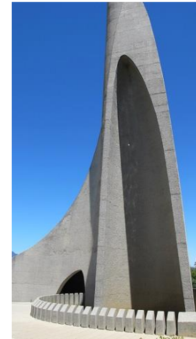
Figure 220 Taalmonument , secondary silo (photograph by the author)
