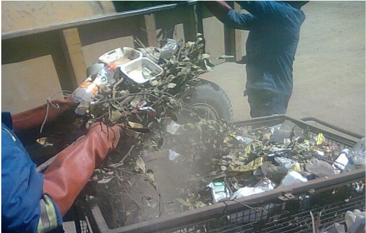
Figure 4.1: Dust generation from loading mixed waste without proper containment bags
