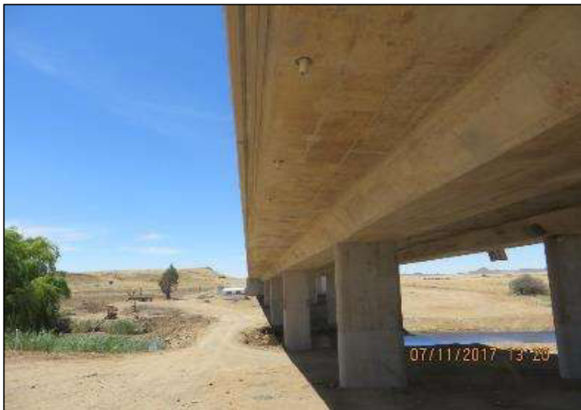
Figure 2.6: Van Zylspruit, 90m integral bridge (Source: Mott Macdonald)
