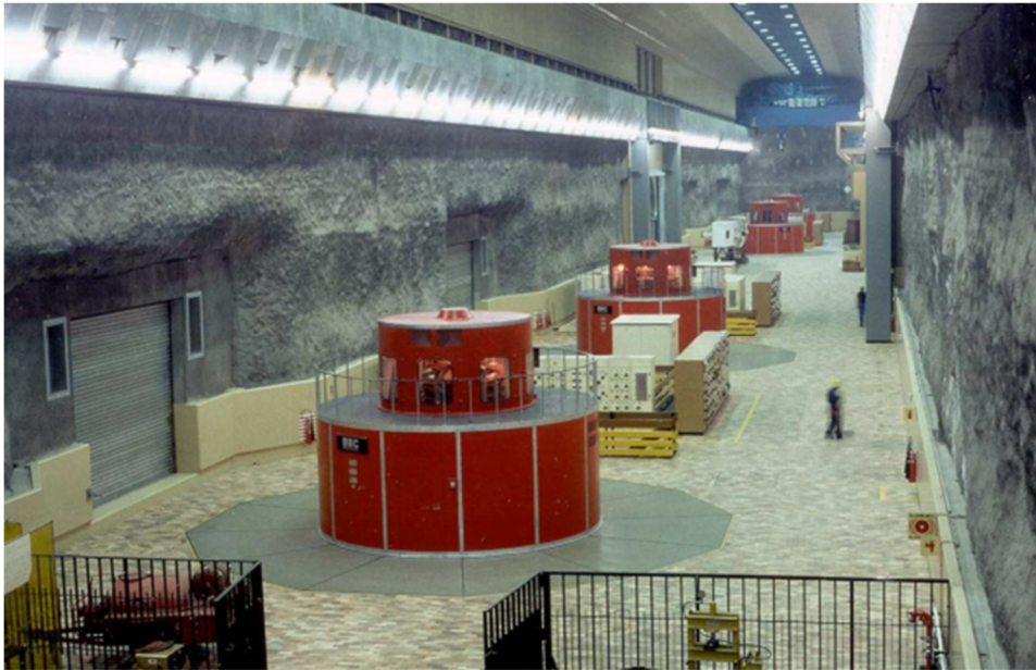
Figure 2-4: Underground machine hall of Drakensberg Pumped Storage Scheme [12]
