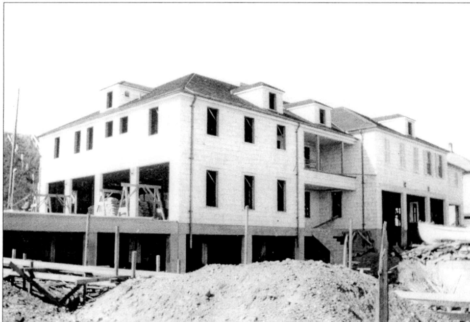
Figure 96. Coquille River Lifeboat Station Under Construction, 1939. Source: U.S. Coast Guard Headquarters (Coquille River File).
