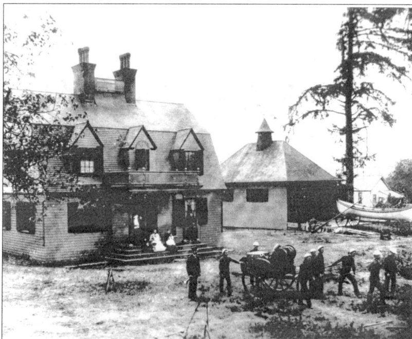
Figure 74. Point Adams Life-Saving Station, Circa 1900. Source: U.S. Coast Guard Headquarters (Point Adams File).
