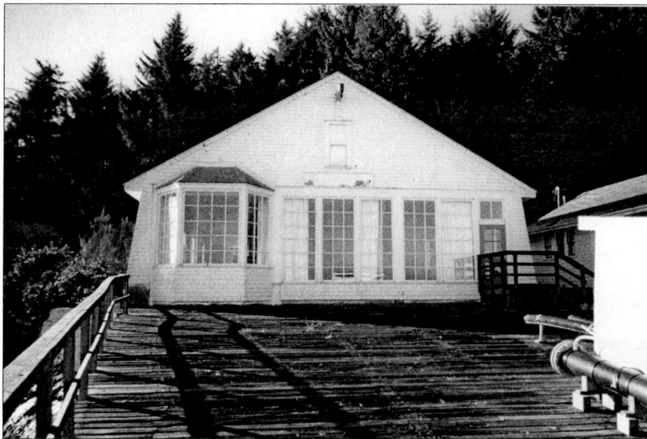
Figure 69. Former Boathouse and Launchway (1915), Coos Bay Lifeboat Station, 1999. Source: Author.
