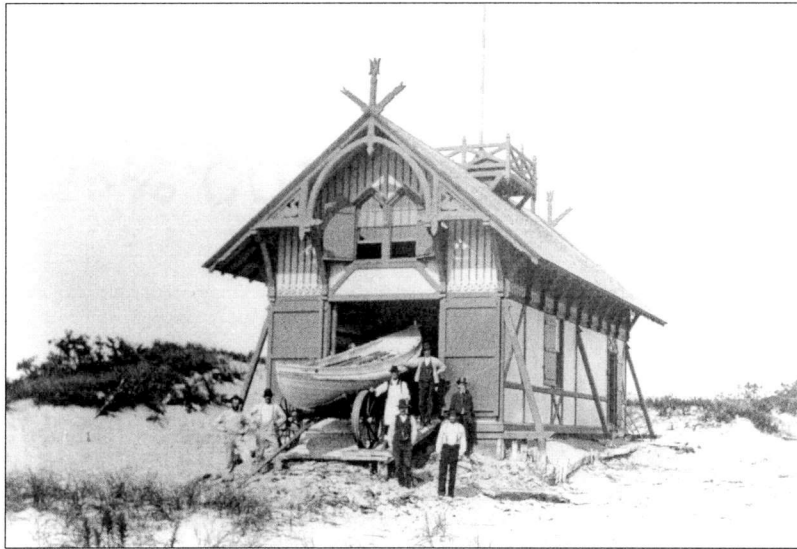
Figure 33. Plum Island Life-Saving Station (Chandler, 1873-74), Massachusetts, an 1874-Type Station. Source: U.S. Coast Guard Headquarters (Life-Saving Service: Stations and Architecture File).
