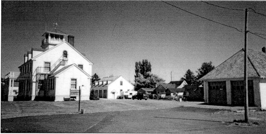
Figure 82. Decommissioned Point Adams Lifeboat Station Complex, 1997. Source: Author.
