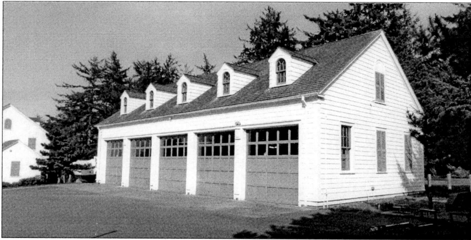
Figure 113. Equipment Building at Umpqua River Lifeboat Station, 1991. Source: Oregon State Historic Preservation Office (Umpqua River Coast Guard Station File).
