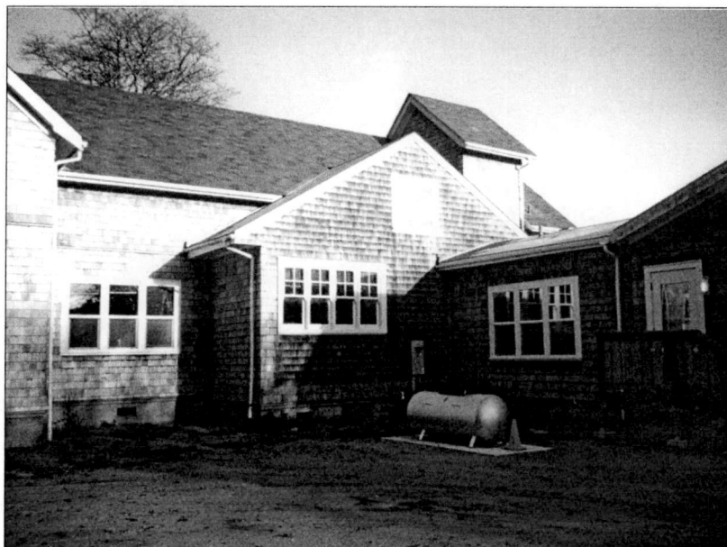
Figure 71. Former Keeper's Dwelling (1915), Coos Bay Lifeboat Station, 1999. Source: Author.
