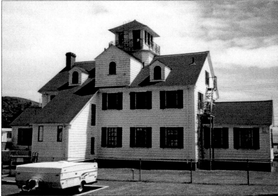
Figure 155. Rear Elevation, Tillamook Bay Lifeboat Station, 1997. Source: Author.
