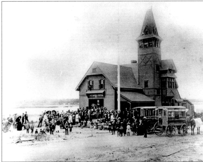
Figure 35. Deal Life-Saving Station (Pelz, 1882-83) in New Jersey. Source: U.S. Coast Guard Headquarters (Life-Saving Service: Stations and Architecture File).
