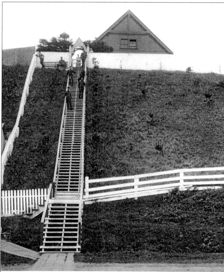
Figure 89. Coquille River Life-Saving Station Staircase to Station House, Circa 1910. Source: Bandon Historical Society (BHS #1559).
