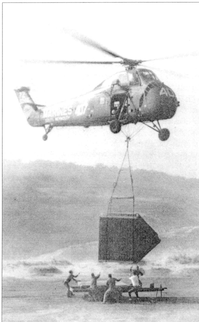
Figure 186. Marine Helicopter Moving Halfway House at Mystic Seaport in 1968. Source: Curtis, Moving Historic Buildings .
