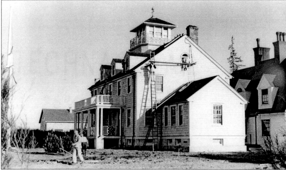
Figure 78. New Point Adams Coast Guard Station, 1939. Source: U.S. Coast Guard Headquarters (Point Adams File).
