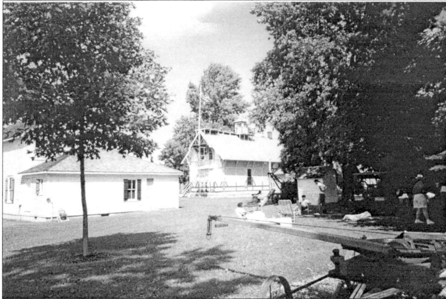
Figure 187. Pointe Aux Barques Life-Saving Station (1875-76) in New Context at Huron City Museum, Huron City, Michigan, 1997. Source: Author.
