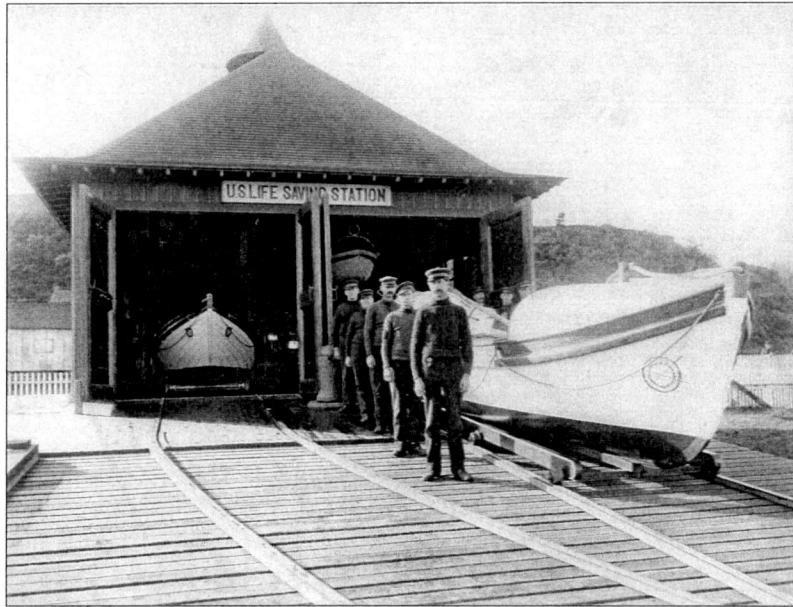
Figure 88. Coquille River Life-Saving Station Crew with Lifeboat, Circa 1912. Source: Bandon Historical Society (BHS #34).
