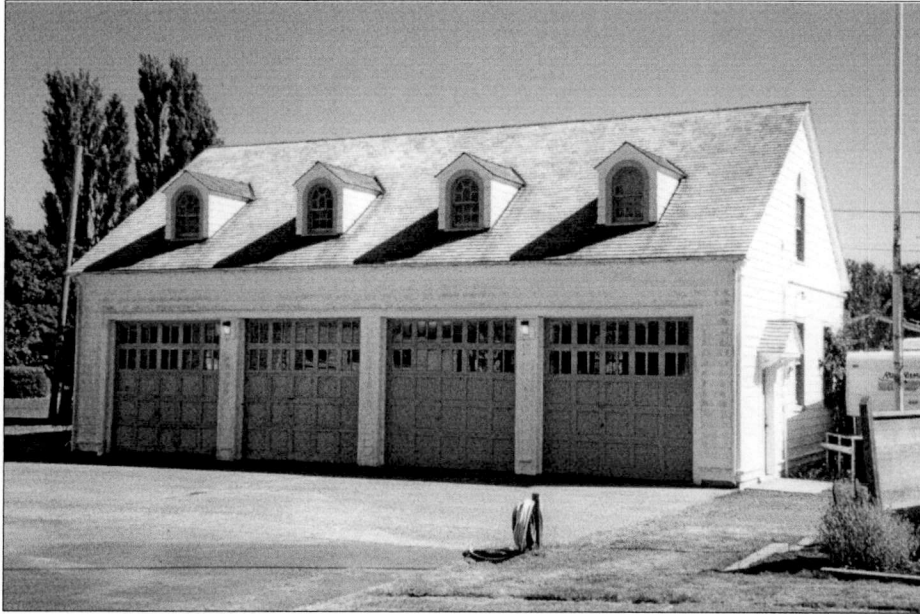
Figure 81. Equipment Building (1939) at Point Adams Lifeboat Station, 1997. Source: Author.
