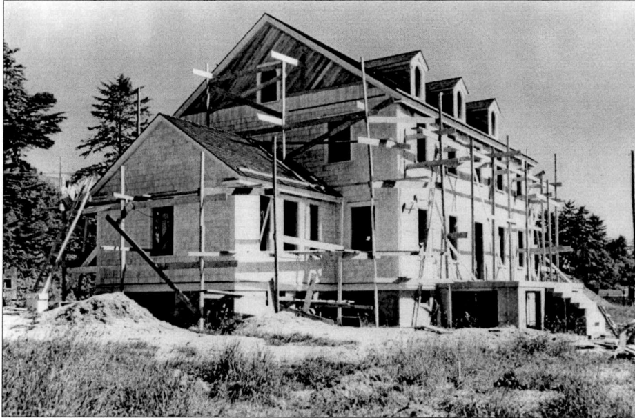
Figure 137. Yaquina Bay Station Under Construction, 1949. Source: U.S. Coast Guard Headquarters (Yaquina Bay File).
