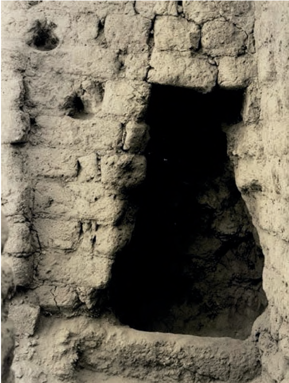
Fig. 5 - Detail of the kiln of the deipneterion . Courtesy of MSA.
