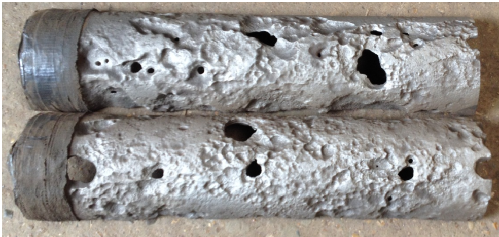
Figure 2.8 - Split section of 4" diameter distribution main illustrating the spread of corrosion and the amount of metal that can be lost to the graphitic corrosion process: (a) before shot-blasting and (b) after shot blasting. After Rainer et al. (2017).
