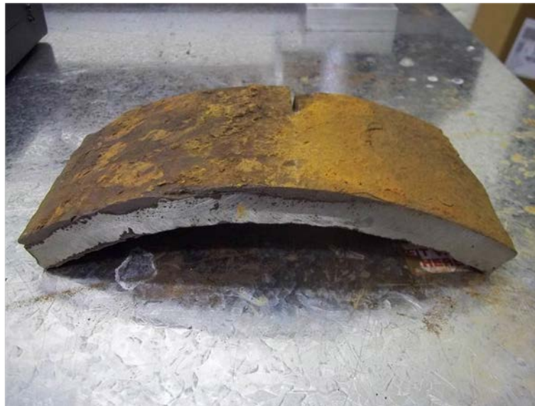
Figure 5.11 - Sample of cast iron trunk main with graphitised layer
