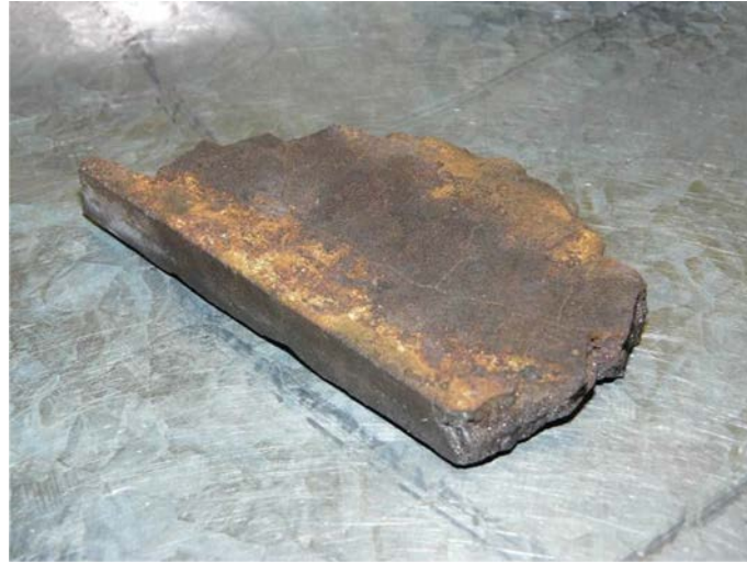
Figure 5.10 - Sample of graphitisation removed from a corroded main
