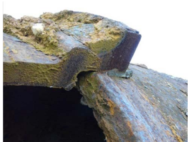
Figure 4. 3 - Barriers to NDE on cast iron trunk main: (a) surface encrustation and (b) variable geometry.
